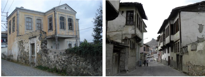
Figure 3. Walls separating the street and the garden and ground floors closed to the outside (E. S. Akin Archive)
