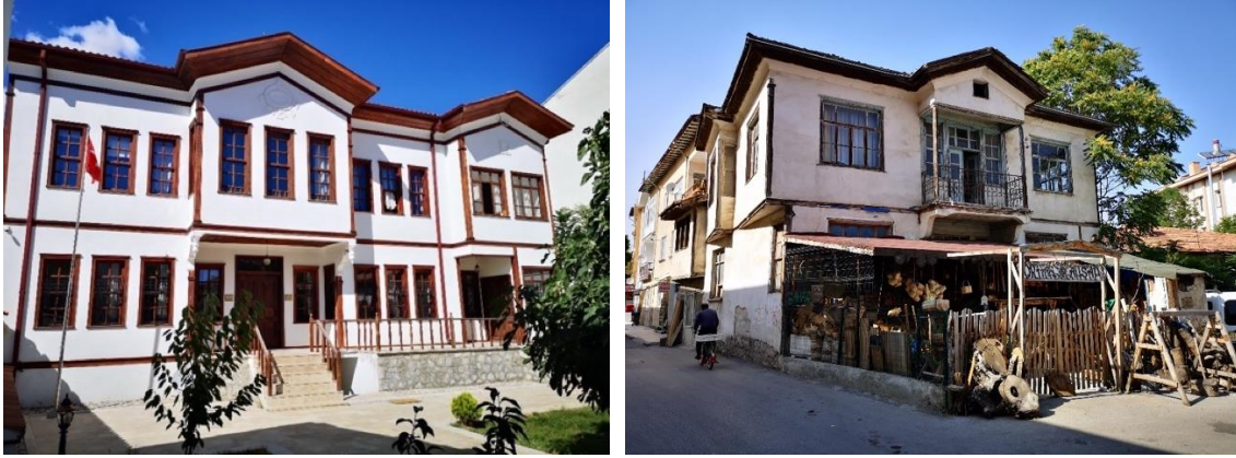
Figure 17. Bilaller Mansion (left), which was restored and functioned as the Provincial Directorate of Culture and Tourism, and the house, which was not restored and whose ground floor was used as a wooden shop and the upper floor was used as a warehouse, Üçtutlar Mahallesi No: 2 (F. Karahan Archive)
