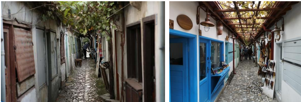
Figure 12. Dikiciler Arasta and Eskiciler street before restoration (left) (Habercim19 Archive) and its current state (right) (F. Karahan Archive)
