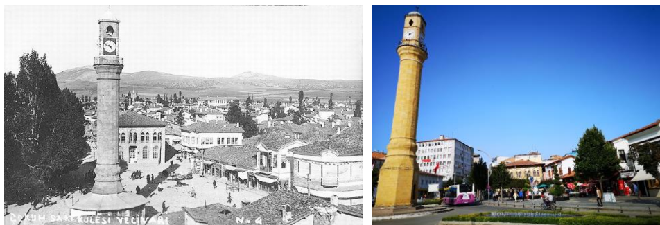
Figure 6. Traditional urban texture with identity as seen in the old photograph of Corum city center [17]
